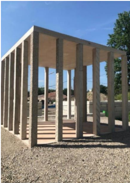
Figure 2: Small-scale action in Munich: sample pavilion of R-concrete (City of Munich)
