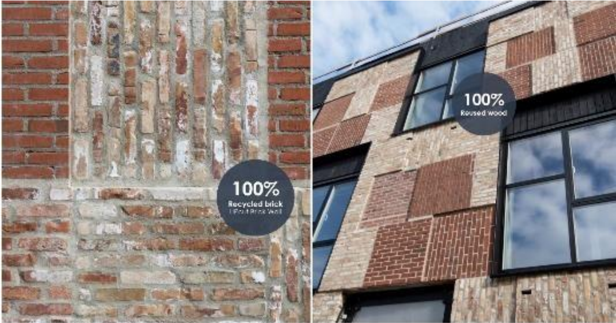
Figure 6: Building facade with secondary bricks in Denmark
