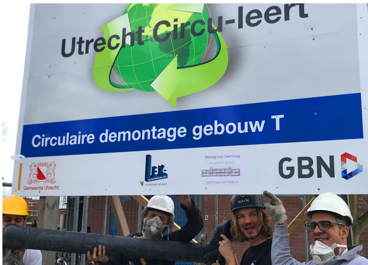
Circular demolition of the RotoSmeets & T buildings at Merwedekanaalzone, Utrecht
